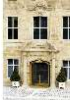
BayO.I, Opernhausmuseum, Portal/Eingang, DI026278, BSV
