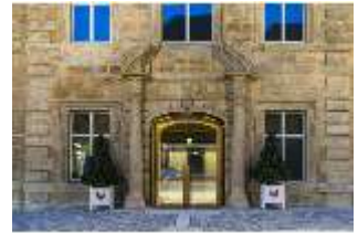
BayO.I, Opernhausmuseum, Portal/Eingang, DI026492, BSV
