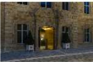
BayO.I, Opernhausmuseum, Portal/Eingang, DI026493, BSV
